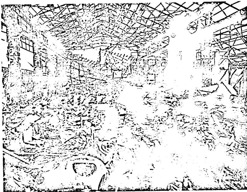
FIGURE 301.—Interior of foundry building of Mitsubishi Steel and Arms Works shown in figure 299, about \frac{1}{4} mile from zero point, showing chaos created by detonation, with torpedo molds and equipment thrown in all directions. Frame of building is grossly distorted, and its corrugated iron covering has disappeared.
