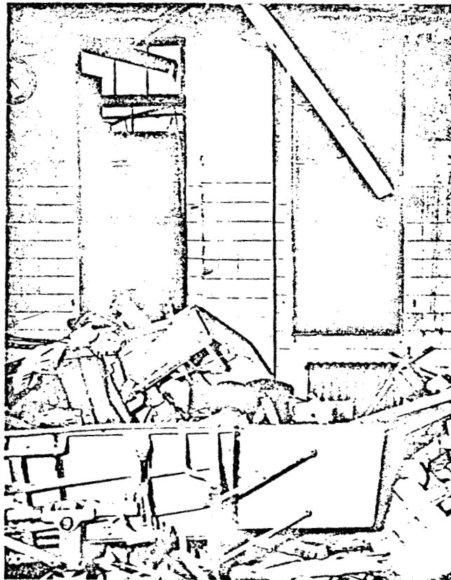
FIGURE 304.—Urology clinic in medical school at Nagasaki 6 weeks after detonation of bomb, showing disarrangement of furniture and equipment. Ceiling soundproofing is torn off and scorched by fire that apparently started at base of ceiling fixture and was caused by violent oscillations of lamp and short circuit at its base. Fuses had been replaced by coins, and the short circuit ignited the corn-husk soundproofing which did not, however, burn sufficiently to drop embers on floor and start fires which occurred for this reason in other parts of the building. No bodies were found in this clinic.
