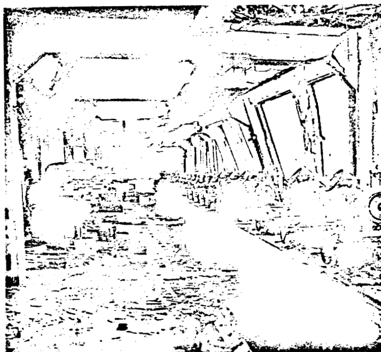
FIGURE 303.—Interior of building shown in figure 302, with front wall displaced inward and window frames gone. There was no fire. Room has been cleaned by Japanese Army workers, but bench lathes exposed to weather are no longer usable. No information could be obtained on casualties among the workers who, if they were standing at workbench shown, were facing the blast.
