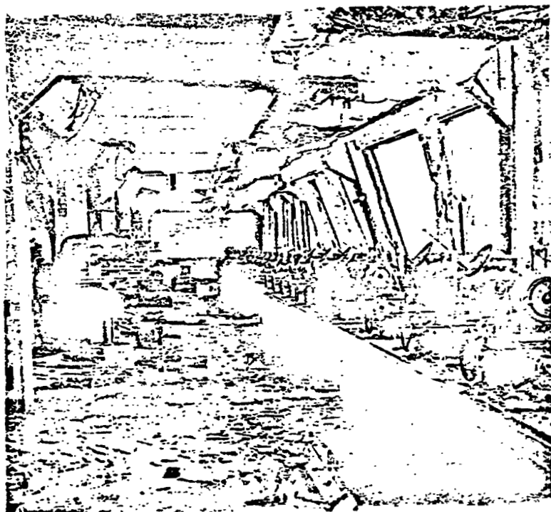
FIGURE 303.—Interior of building shown in figure 302, with front wall displaced inward and window frames gone. There was no fire. Room has been cleaned by Japanese Army workers, but bench lathes exposed to weather are no longer usable. No information could be obtained on casualties among the workers who, if they were standing at workbench shown, were facing the blast.
