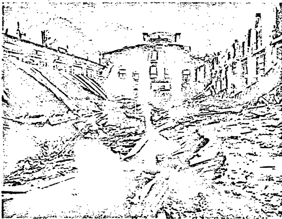
FIGURE 300.—Modern pattern works of German design at Nagasaki detonation of atomic bomb. The roof had collapsed upon about 300 workers in this building and in the similar building next to it.
