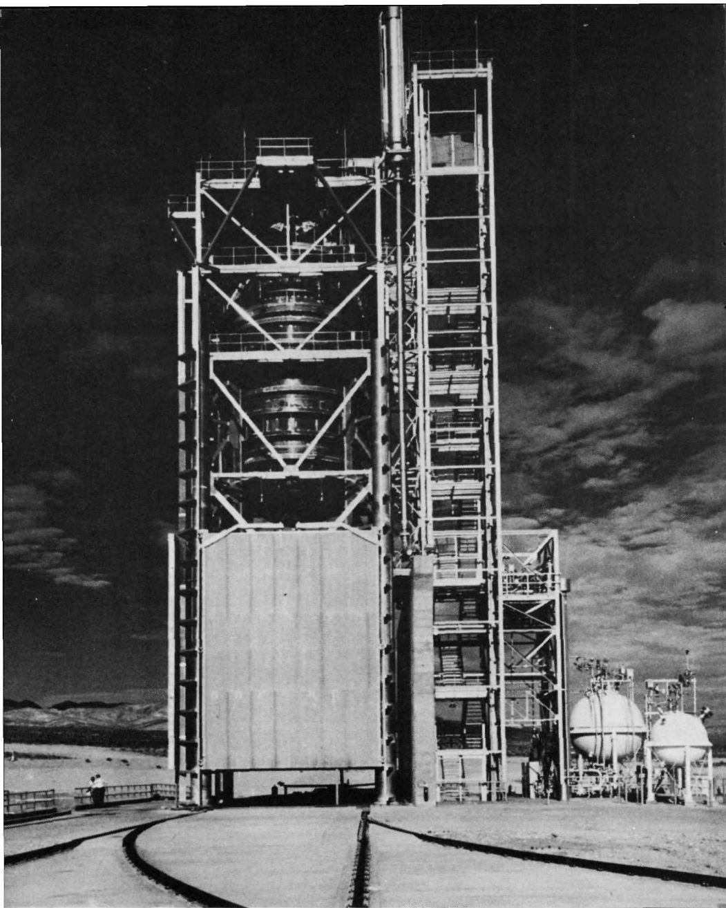
Engine Test Stand 1 (ETS-1), 140 feet (43 m) high, where NERVA engines are tested at NRDS. White spheres at right are dewars for liquid hydrogen and liquid oxygen. The hot exhaust rushes down through a duct to the deflector, at left, below where men are standing. Tracks permit railroad to bring in engine and shields.
