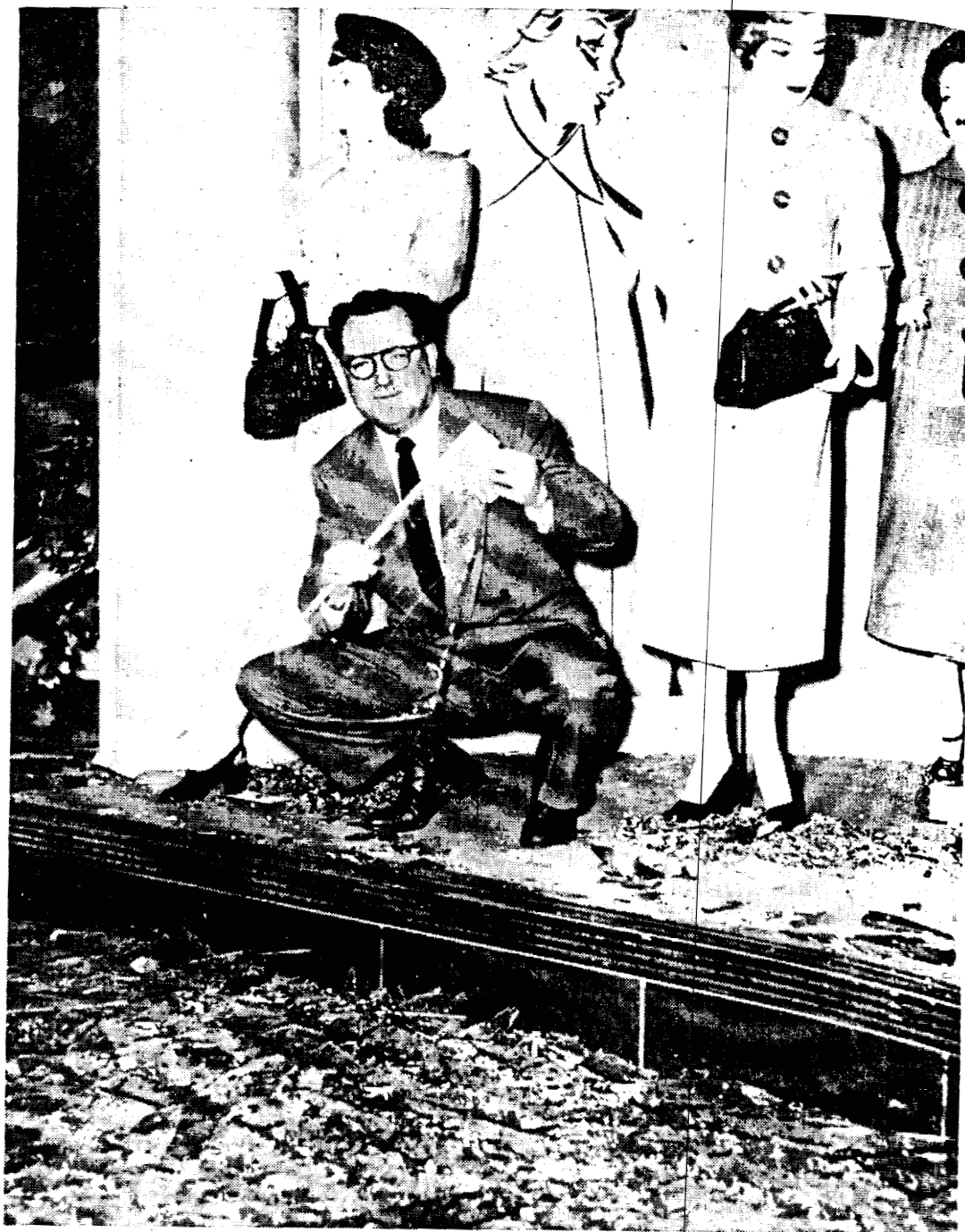
A downtown Las Vegas window, showing how the glass was sucked out by the rarefaction wave, rather than pushed in by the compression wave resulting from the November 1, 1951, nuclear test at the Nevada Proving Ground.
