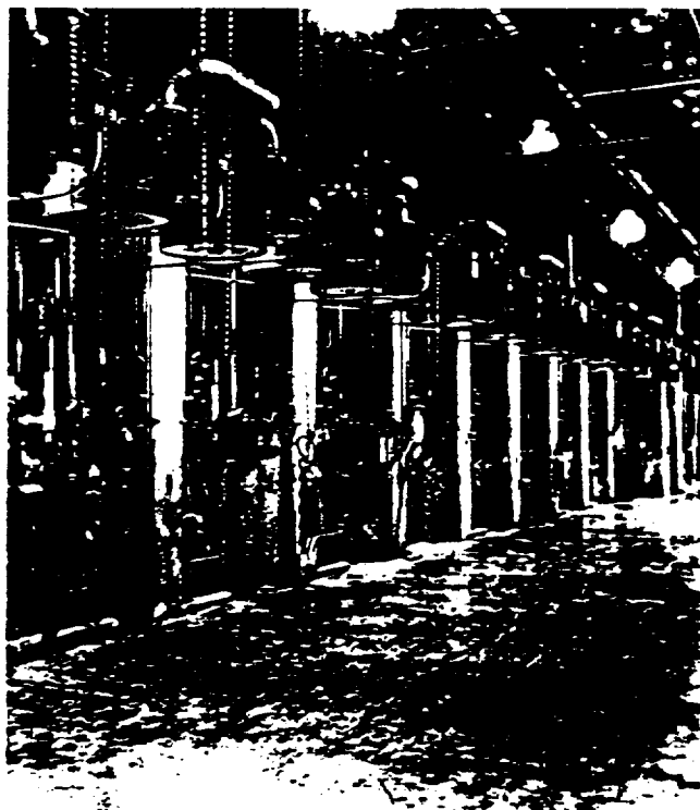
A vast bank of diffusion vacuum pumps operated underneath the alpha calutron racetrack to free the tanks of air.
