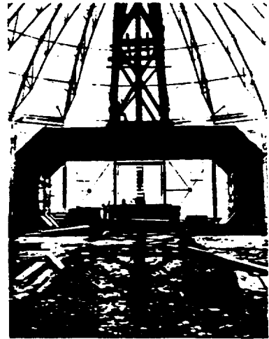
The magnet yoke for the 184-inch cyclotron during construction.
